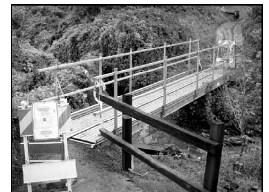
High water in San Vicente Creek is eroding the foundations of the footbridge.
