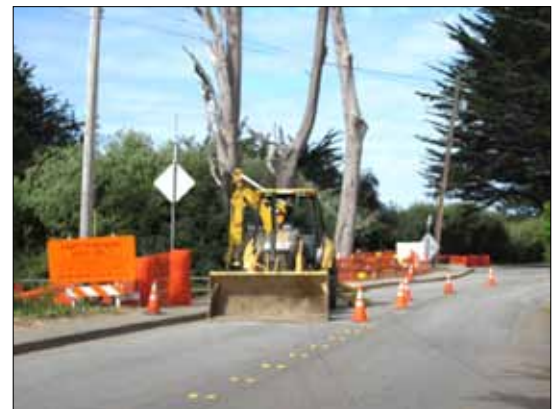
Work progresses on North Lake Street.
