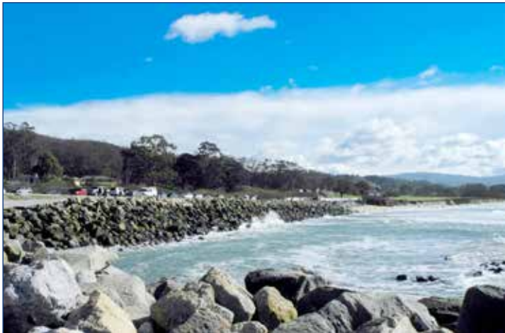
Dramatic erosion south of the breakwater
