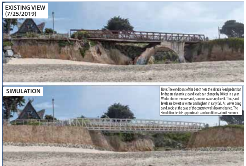
Mirada Bridge, existing and simulation of possible future structure Photo courtesy of Coastside Buzz
