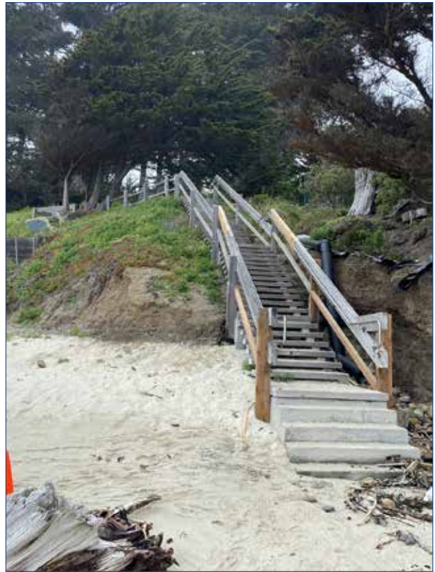
Repaired Seal Cove stairs, photo: Martie Sautter
