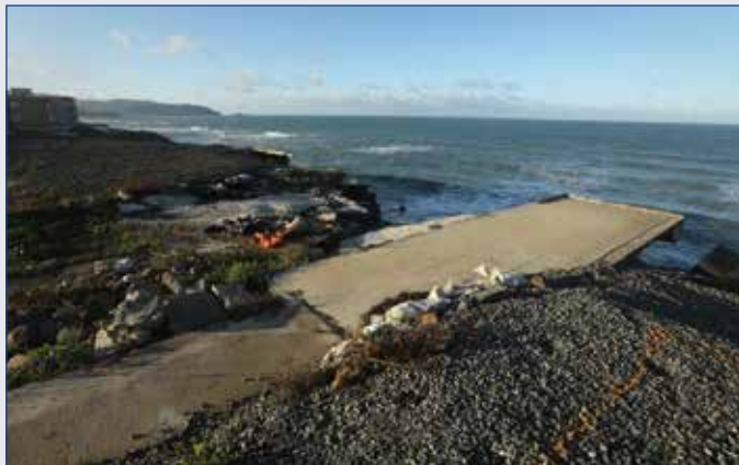
Along Esplanade Avenue in Pacifica, a walkway is all that's left of an apartment building. (Carolyn Cole / Los Angeles Times)
